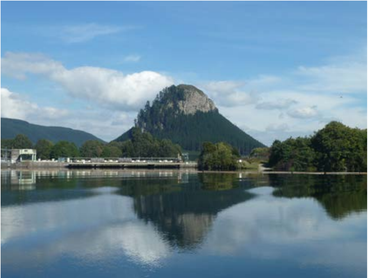
POHATURA & LAKE ATIAMURI WITH MRP HYDRO STATION. Pohaturua is a key landmark or Pou for Raukawa and is seen from Lake Atiamuri
