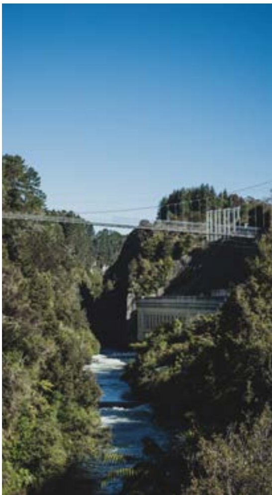
Arapuni Power Station on the Waikato River with Waikato River Trails Swingbridge
