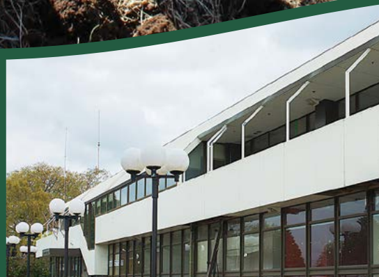
New Premises Underway
