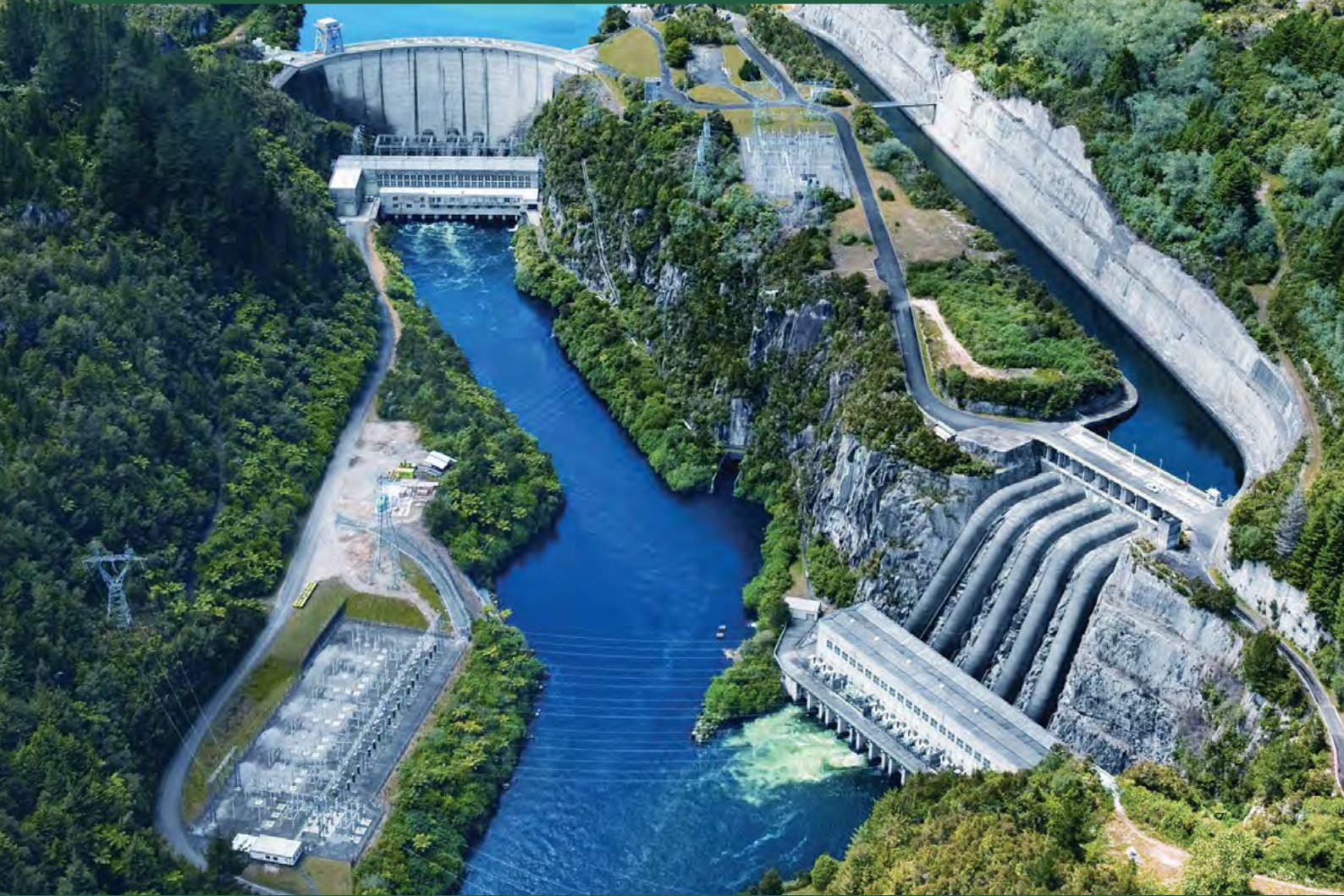
Maraetai Dam and Power Station.
